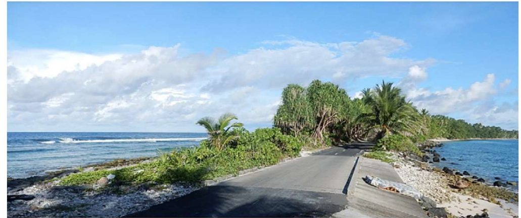
Coastal erosion in Tuvalu. Photo: Michael Coghlan
